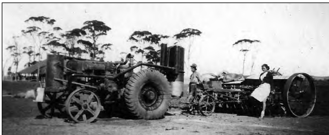
1932 Case tractor fitted with a Hewitt gas producer (Jack McCorry and Clarice Herbert) Photo courtesy of Bob Herbert
