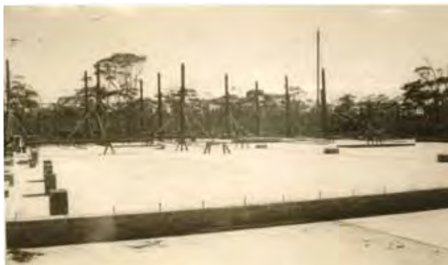
Foundations and partially erected columns, No.1 Workshop (Picture taken by Lt. Col. H.B. Jarvis)
